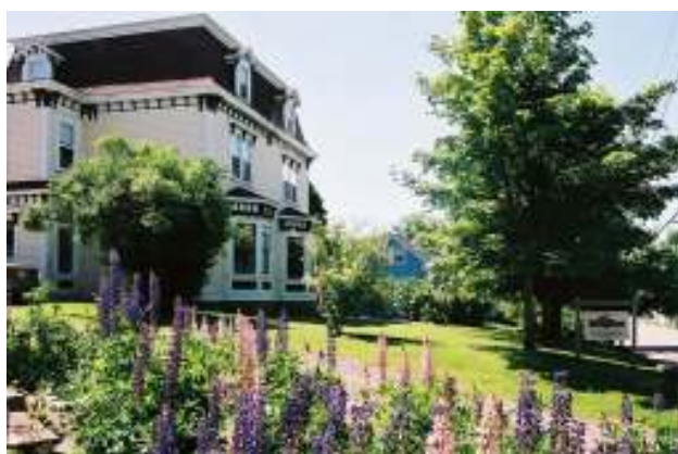
"The Maples" as restored by WHS
