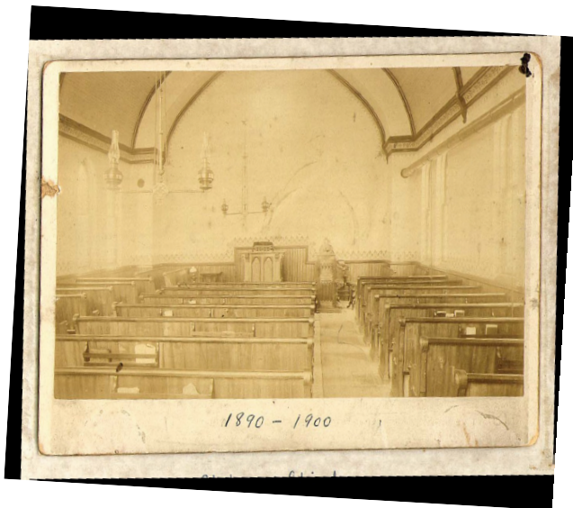
St. James Interior ca. 1900
